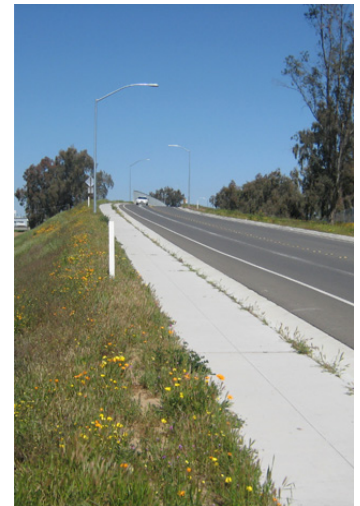
Measure T Tier 1 project: Gateway Drive overcrossing at State Route 99.
